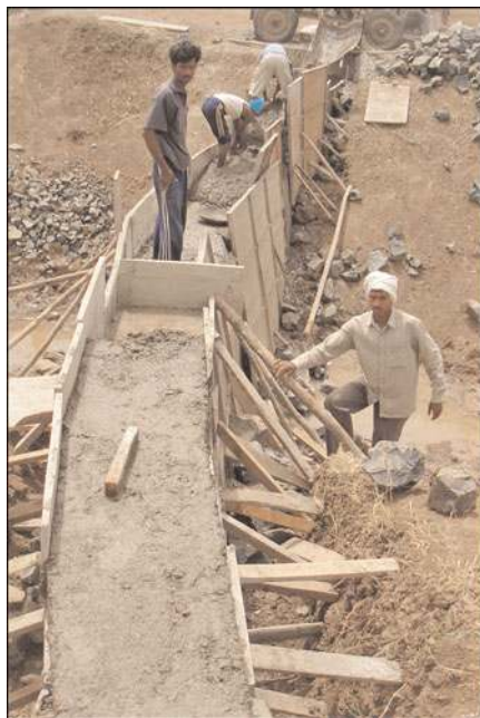
FIGURE 7.2 Check dam: a work in progress.
