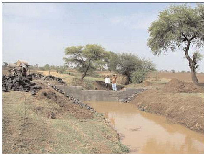
FIGURE 7.3 Check dam: work is completed.
